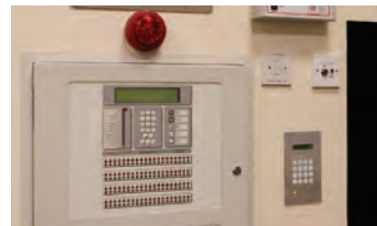
Fire Alarm Systems
